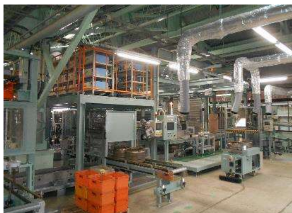
Renewal of in-house plating equipment to improve plating quality and enhance production of screw products
