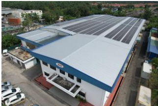
Solar panels (Subsidiary in Malaysia)
