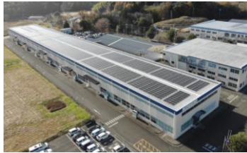
Solar Panels (Ayabe Assembly Machinery Plant) →Achieved 100% Green Energy
